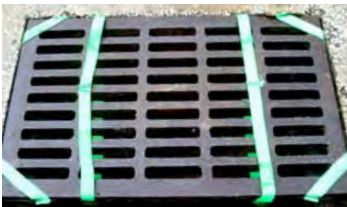
Step 3: Affix the corner webbing over each of the grate's four corners one at a time.
