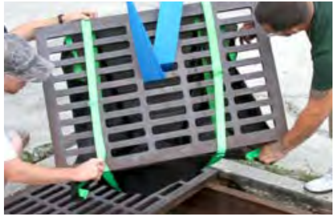
Step 2: Slip the webbing over the ends of the grate one side at a time.
