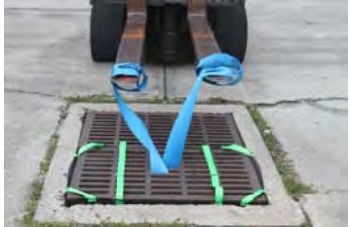
Step 4: Replace the grate.
