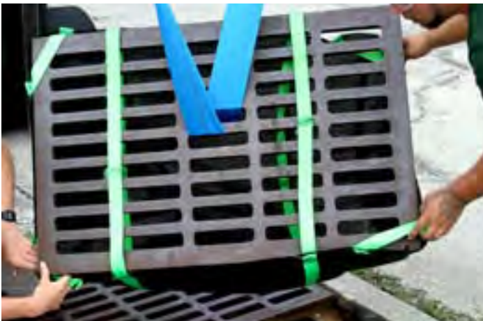
Step 3: Affix the corner webbing over each of the grate's four corners one at a time.
