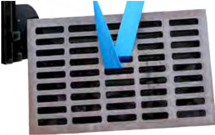
Step 1: Lift the grate using a grate hook or proper mechanical equipment.
