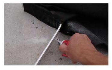
Step 6: Fasten the first aluminum angle bracket with tapcons.
