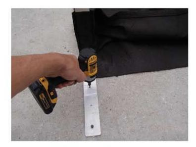
Step 7: Pull the bag taught and align the second bracket. Repeat steps 4-6. Once complete, both brackets should be fully secured to the concrete.
