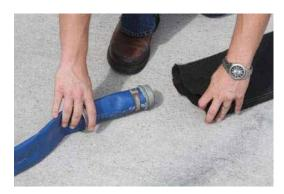
Step 3. Insert the pipe, hose or discharge into the sock. The clamp should be kept far back on the hose/pipe so that it does not enter the sock area.
