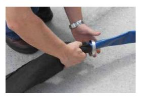
Step 4. Squeeze the dewatering sock tightly to the pipe/hose. Slide the clamp over the sock so that it is covering both the sock and the hose/pipe.
