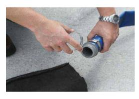
**Step 2.** Slide loosened clamp over a pipe or hose.
