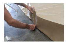
Once all the angles have been inserted, sit the walls of berm up to complete your containment area.
